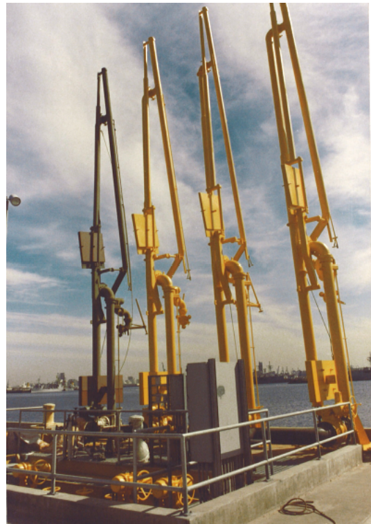
channel of Los Angeles harbor to the new tank farm at the Navy Mole on Terminal in Long Beach.
